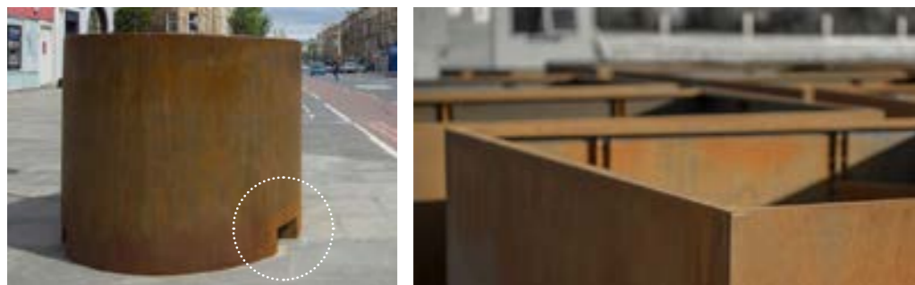
Forklift slots fabricated for mobile planters/additional flexibility
