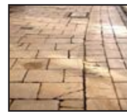
Buff Marshall's Saxon paving on Micklegate incorporating a pavement widening
