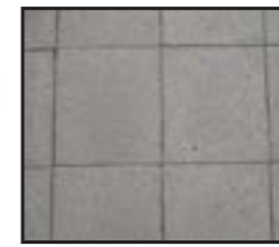
Grey Marshall's Perfecta paving on Lendal Bridge laid as a stacked bond
